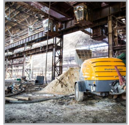
Russia, Ryazan placement of ~100,000 m 2 of screed
