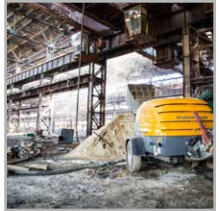
Russia, Ryazan placement of ~ 100,000 m 2 of screed
